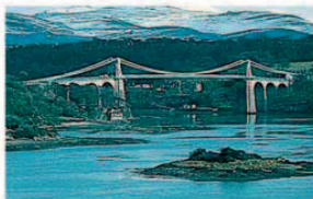
мост most bridge
